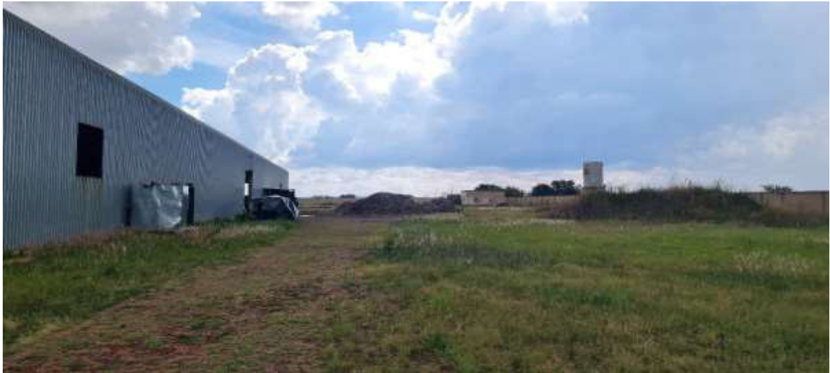
Photo 10 External View of Warehouse / Operational Area
