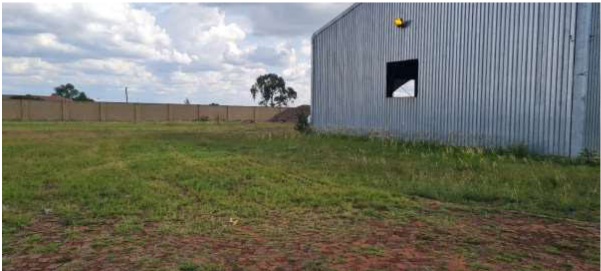
Photo 11: External View of Warehouse / Operational Area
