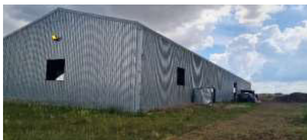
Photo 1: External View of Warehouse
