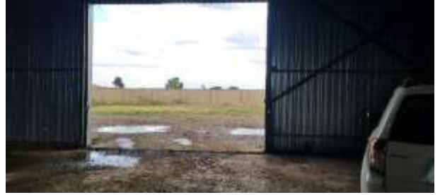
Photo 4: Side Access Point into the Warehouse
