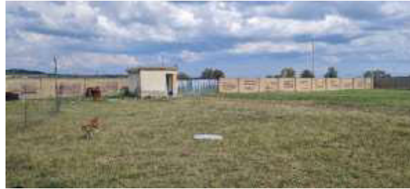
Photo 4: Site fence and access point
