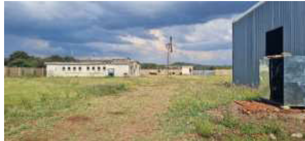
Photo 6: Site office and general site view
