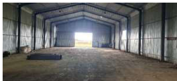
Photo 2: Internal View of Warehouse
