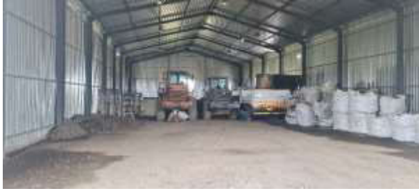
Photo 3: Internal View of Warehouse
