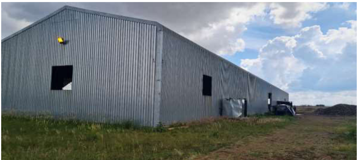
Photo 9: External View of Warehouse / Operational Area
