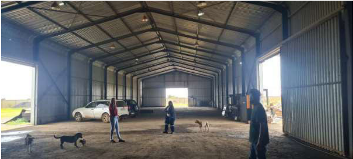
Photo 4: Operational Area – South-east View
