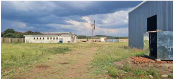
Photo 5: View of On-site Roadway Leading to the Warehouse
