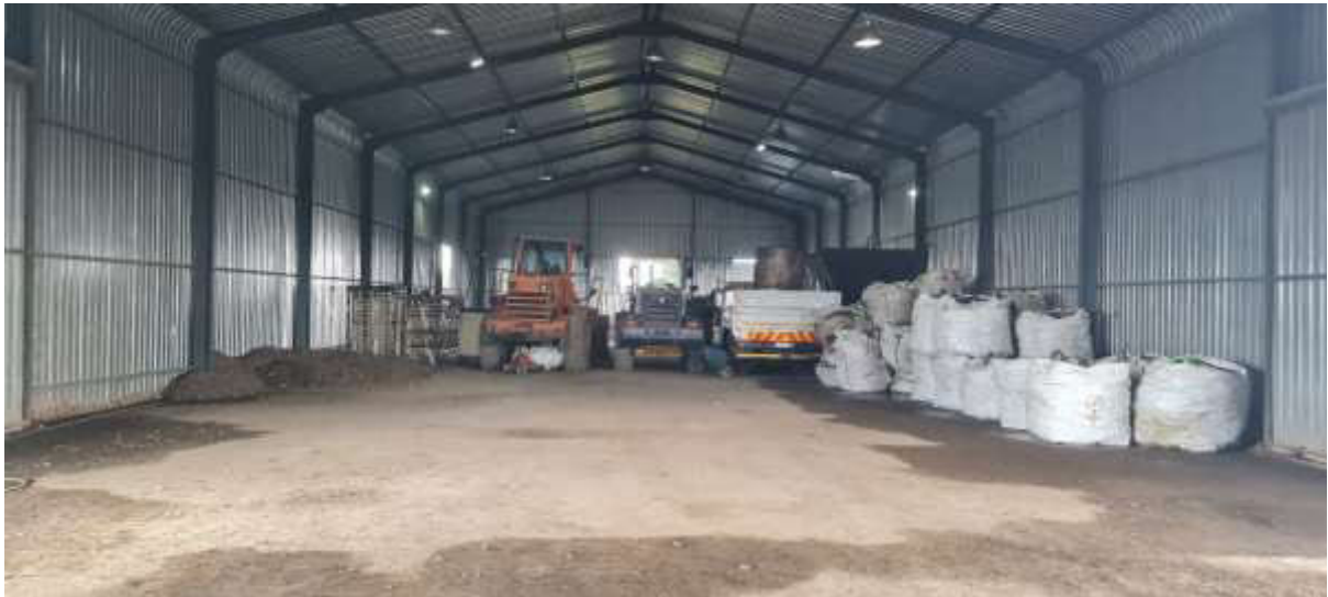
Photo 5: Operational Area - South View
