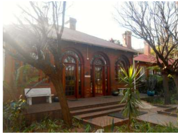
Figure 22. Crown Mines Head Office
