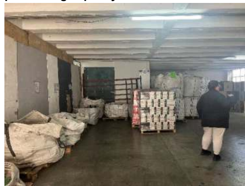
Figure 7. Cemented surfaces inside building.
