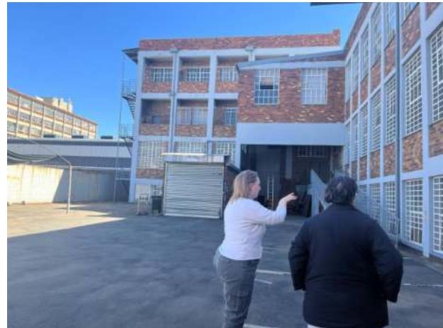
Photo 14: Extension site View of yard
