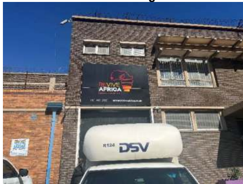
Figure 4. Revive Africa (existing operation) building
