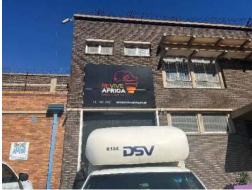
Figure 2. Revive Africa (existing operation) building
