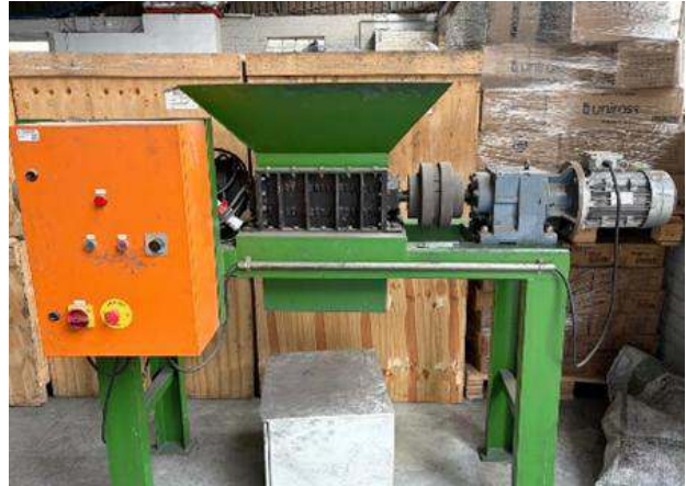
Photo 8: LIB Shredder Station
