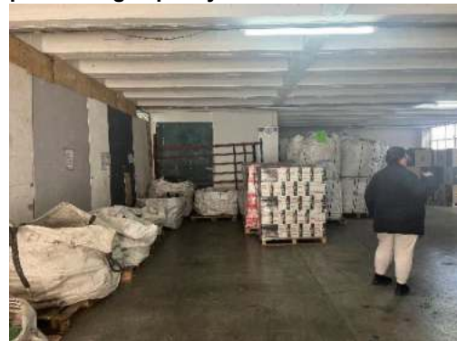
Figure 5. Cemented surfaces inside building.
