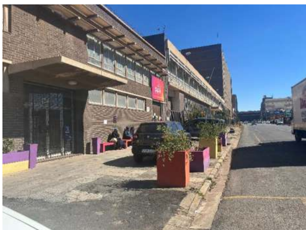
Photo 1: External view of existing site
