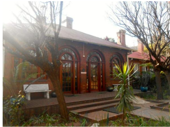
Figure 22. Crown Mines Head Office
