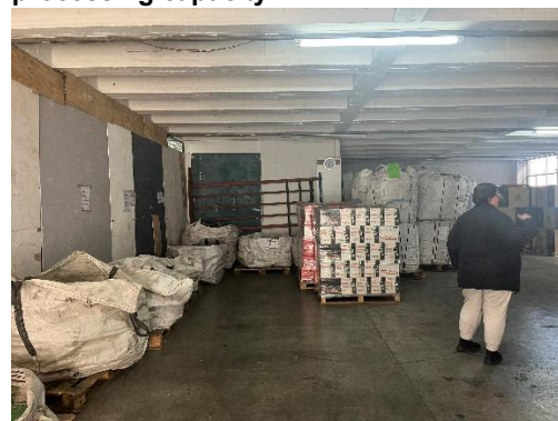
Figure 5. Cemented surfaces inside building.
