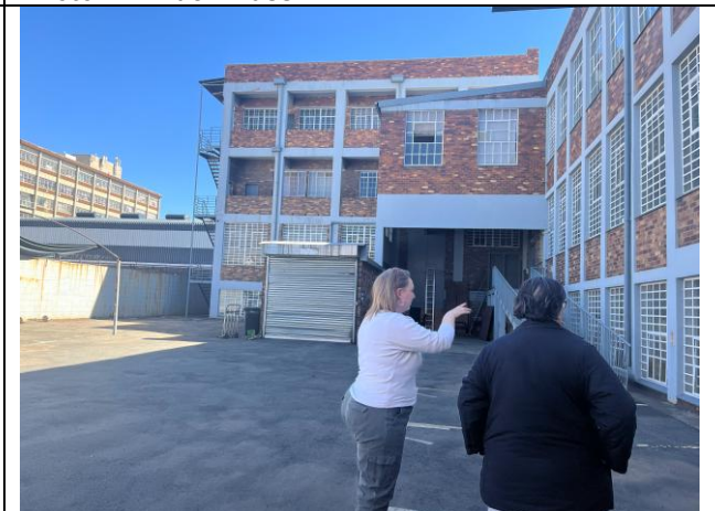
Photo 14: Extension site View of yard
